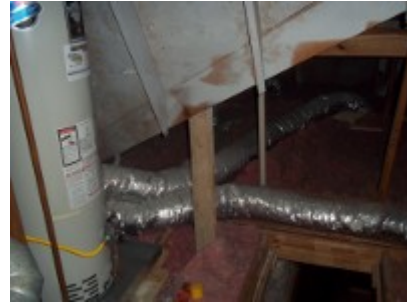
Workspace for water heater lacking ducts on insulation.
