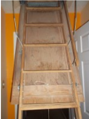
No insulation on door.
