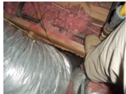
Workspace for water heater lacking ducts on insulation.
