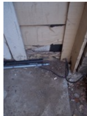
Downspout dumping water down on path.
